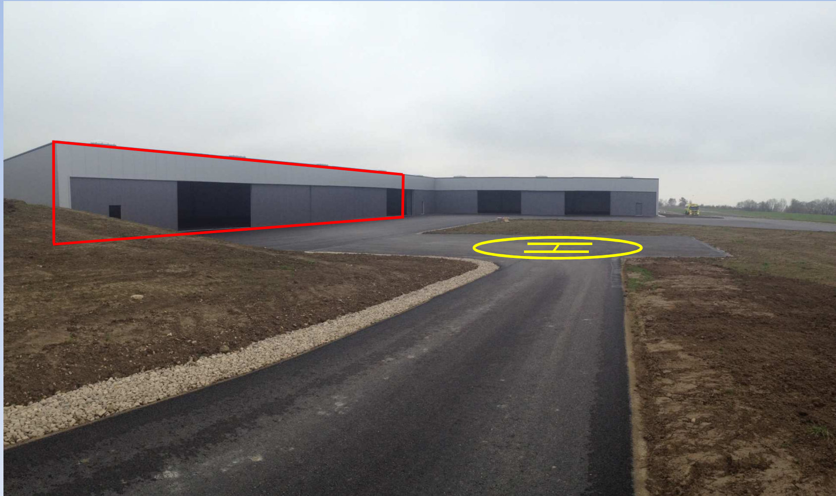
Hangars + helipad Heli-Lausanne
