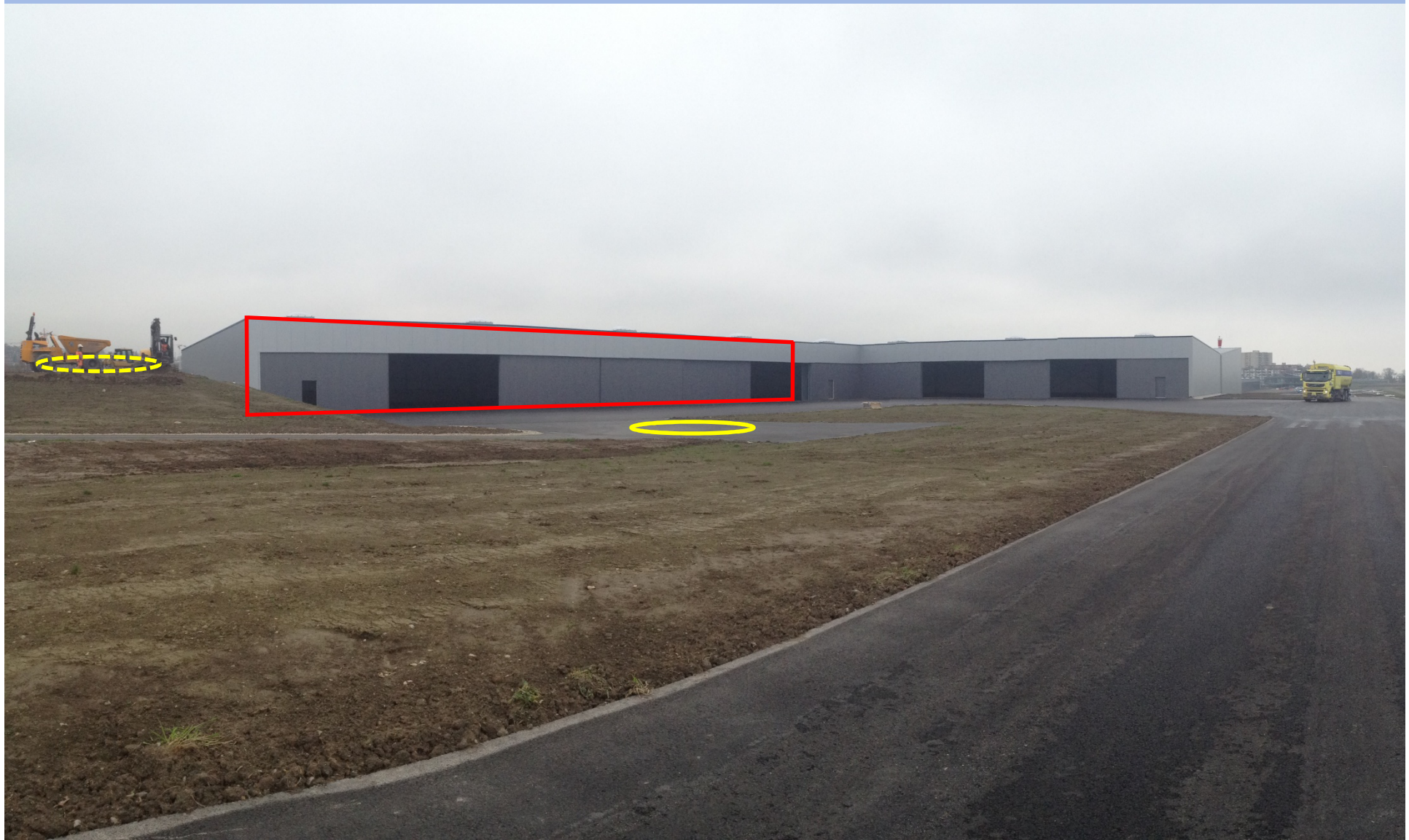
Hangars + helipad Heli-Lausanne
